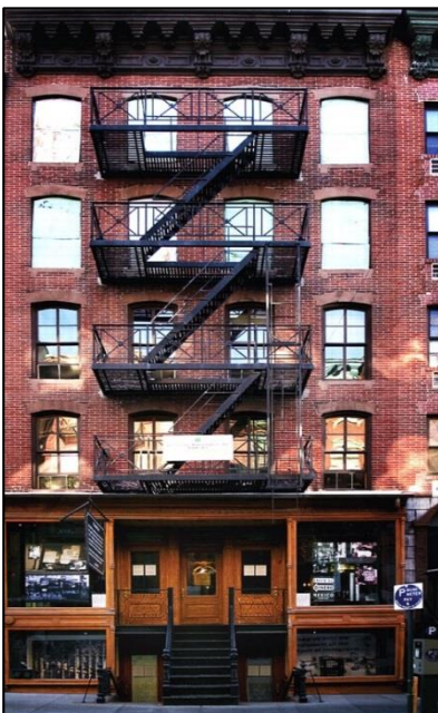
Figure 1: The exterior of the Lower East Side Tenement Museum. The building was constructed using cheap materials and many apartments had no running water.
