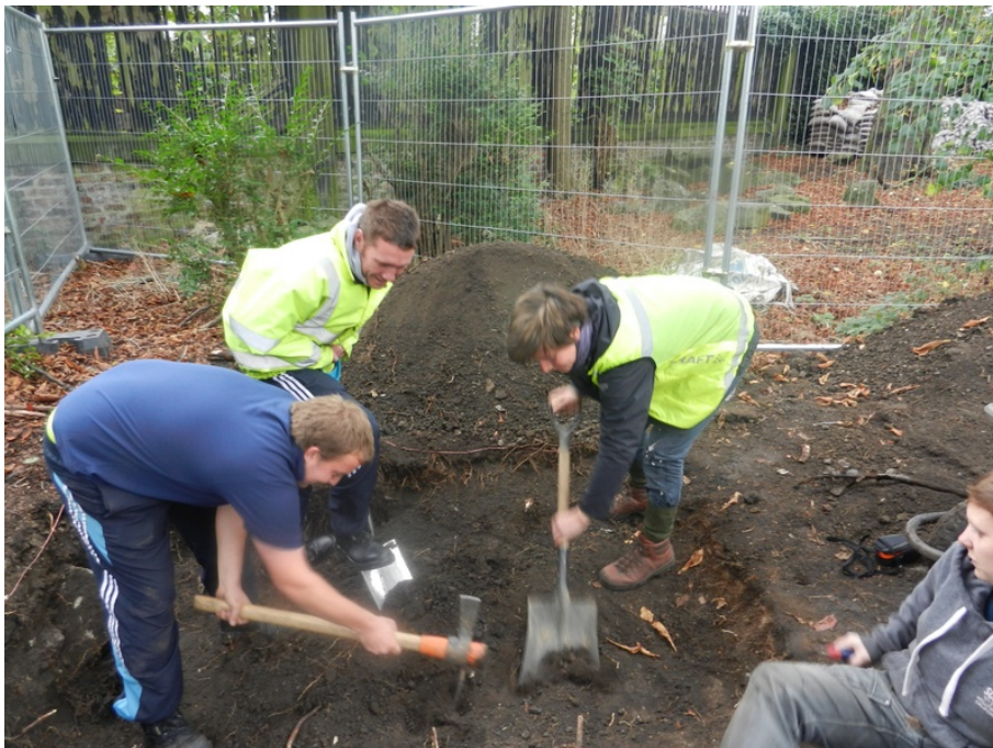
Figure 2 – The team working together on site (Image copyright – Martyn King)
