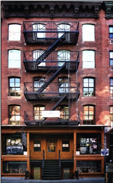
Figure 1: The exterior of the Lower East Side Tenement Museum. The building was constructed using cheap materials and many apartments had no running water. (Image: Fletcher6, Creative Commons, 2012).
