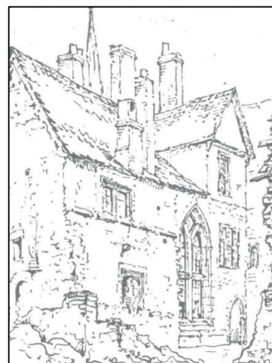
Figure 7. Buckler's sketch of the South West aspect following demolition of the post-medieval wings (Munby 1979, 135).
