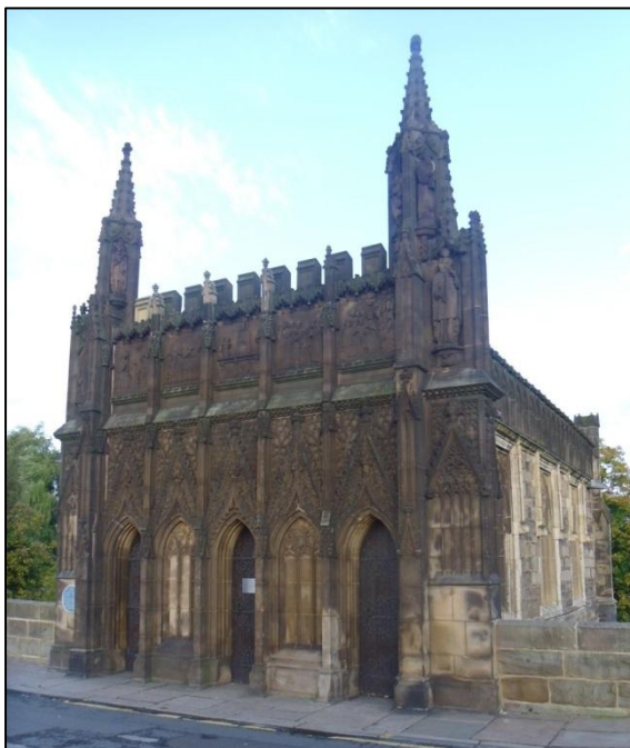
Figure 12. The facade today, much weathered and dirtied by passing traffic, and with small areas of stone replacement evident (authors own).
