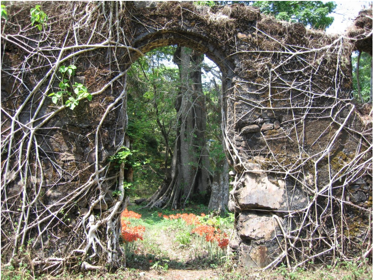
Figure 5: Part of the outer wall and Merchant Dormitory of Bunce Slave Fort (Image Copyright: Andrew Marriott)
