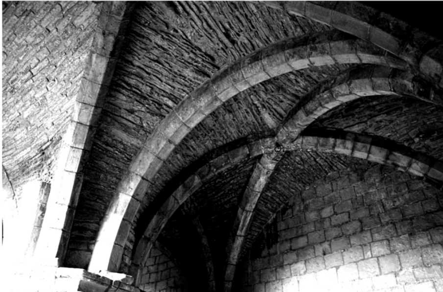
Figure 4. Vaulted ceiling in the basement
