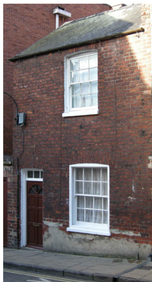
Figure 5: Cumberland street house. Reproduced by kind permission of Richard Green.
